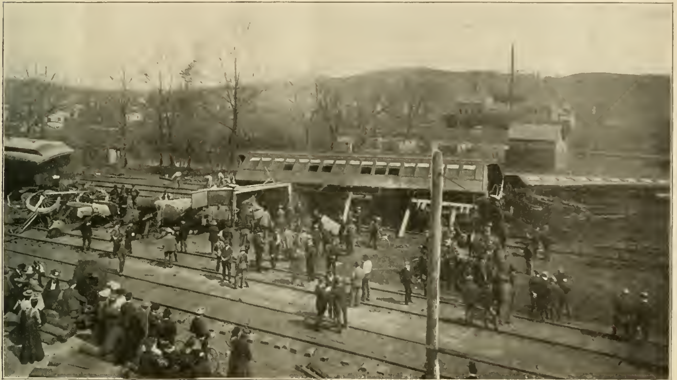
WRECK CAUSED BY BOILER EXPLOSION.
